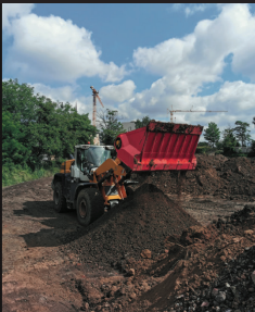
TOPSOIL SCREENING
